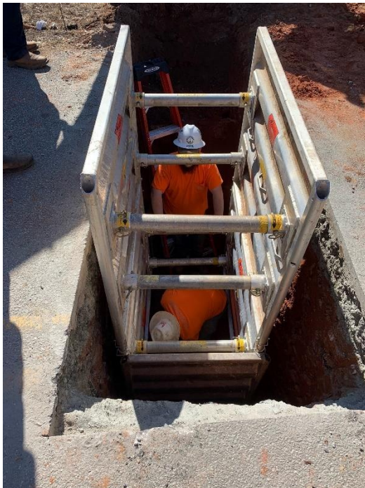
Pictures below: Installing new sewer line on Elizabeth Street utilizing shoring equipment.
